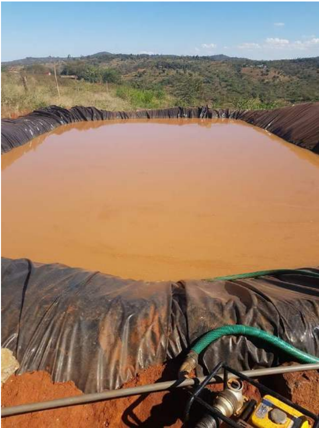
After harvesting water using 0.5mm geomebrane dam liner
